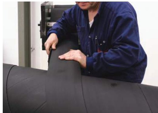
Steel cord reinforcement application
